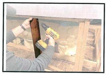
Add additional bracing if necessary, bracing should be no more than 24" apart.
