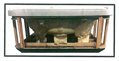
Deactivcate the power to the spa. Remove the old skirting and measure the height. The new skirting will be installed the same way or butting up to the shell
