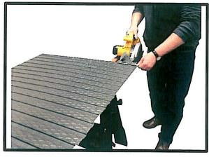
Using a circular saw with a fine tooth blade, cut all 5 panels and both flanges to this height. If using a corded saw, make all cuts a safe distance from the spa.
