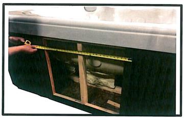
Measure from the outside of each flange and subtract 1" from that measurement. Cut a panel to length using this measurement.
