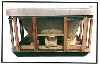
If not already framed in, use a couple of 2x4's to frame out an opening for an equipment service panel. The service panel should be at least 24" in width, but can be wider. One Horizontal support needs to be installed to use as a backer to fasten the service panel to.
